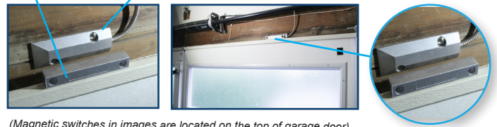
(Magnetic switches in images are located on the top of garage door)
